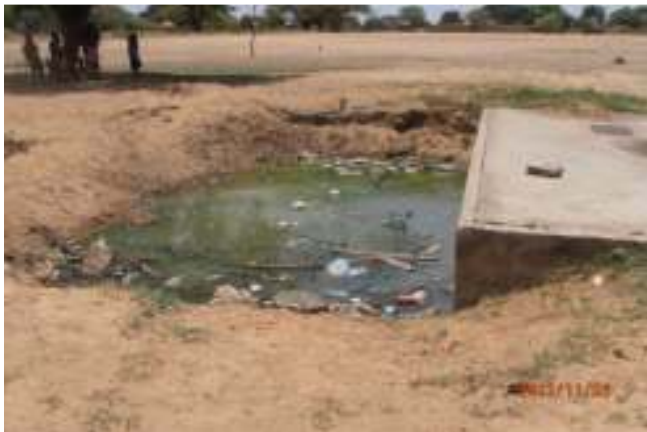
Figure 5 illustrates drainage water due to block sewerage
