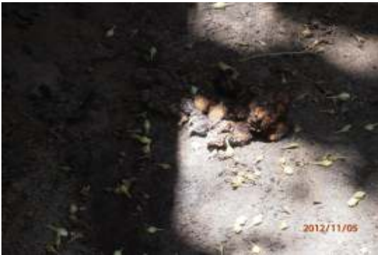
Figure 10 illustrates pit latrine condition for San learners
