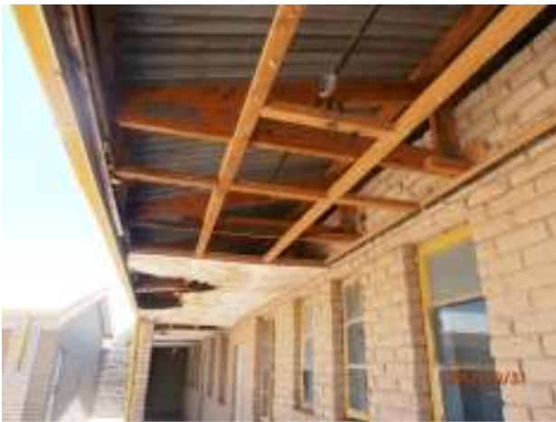
Figure 16 illustrates the Electrical problems
