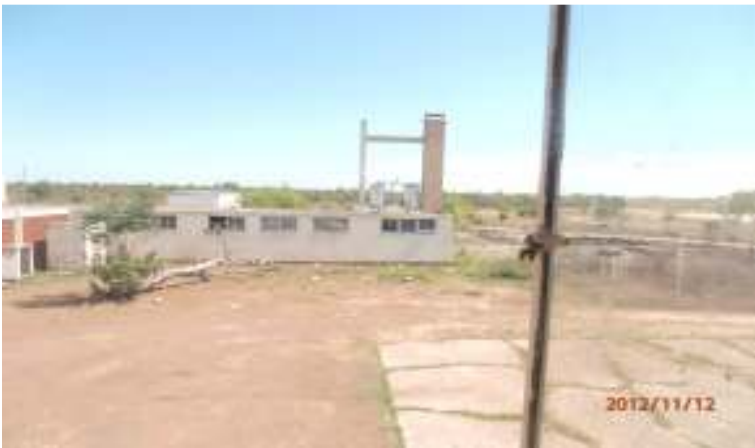
Figure 24 illustrates an unsafe hostel without fence
