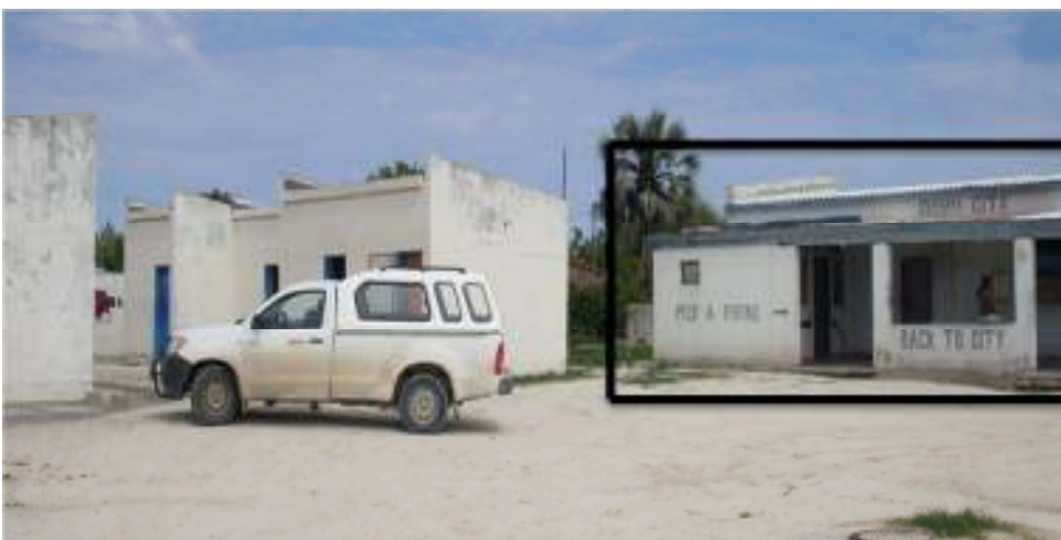
Figure 8: A private bar built on the government premise (police flat) in Ondangwa
