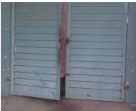
Figure 1(a): A garage rented out in Windhoek
