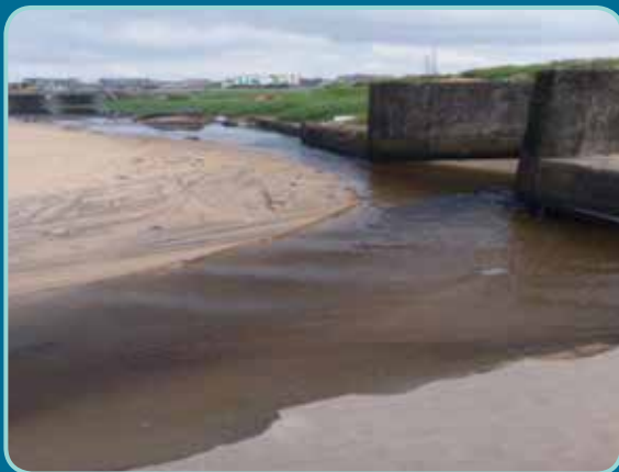
Liberia – General Auditing Commission (GAC) photo: A partial view of culverts conveying sewage and other waste into the ocean in Sonniewein Community, Montserrado County
