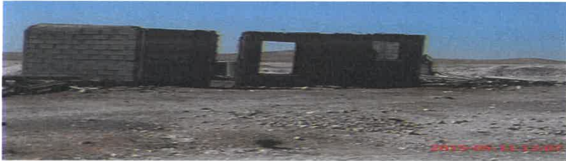
Picture 9: Building not demolished
