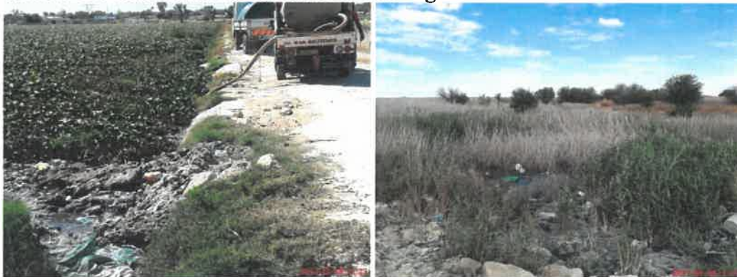
Picture 10: Oxidation Ponds covered with vegetation at Oshakati and Arandis
