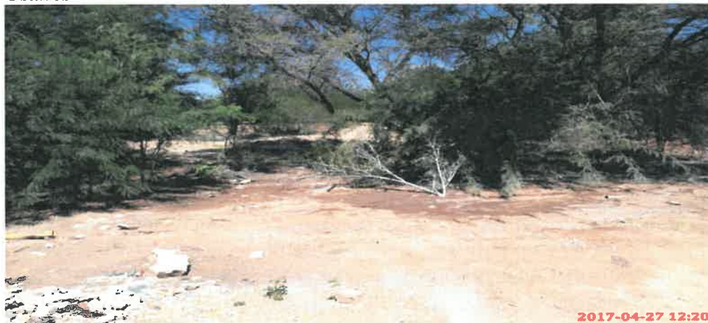
Picture 1: Untreated sewage disposed-off in an open area next to the Oxidation Ponds at Usakos
